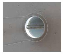
The fire damper cartridge is inserted into a metal ventilation duct of the same diameter, and is held in position by its rubber seal.
